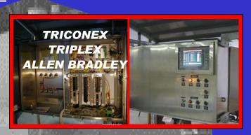
**SIL-bmsTect-2600** can be used in a de-energized to trip or energized to trip applications. For energized to trip applications, the field wires are line supervised to verify and validate the BMS system ability to respond correctly to a shutdown command. Because of the 99% diagnostic coverage factor of its equipment, **SIL-bmsTect-2600** can locate the failure and display the failure on the local CRT or communicate it to the control room via the MODBUS link.
